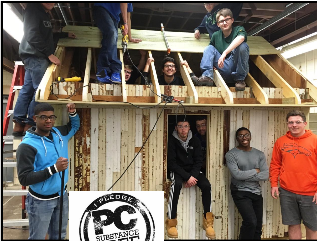
Building Trades Students are Shown Constructing a Storage Shed for the Career Center.
